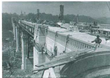
Bloor Street Viaduct Designed / built – 1913 -1918 subway added - 1966
